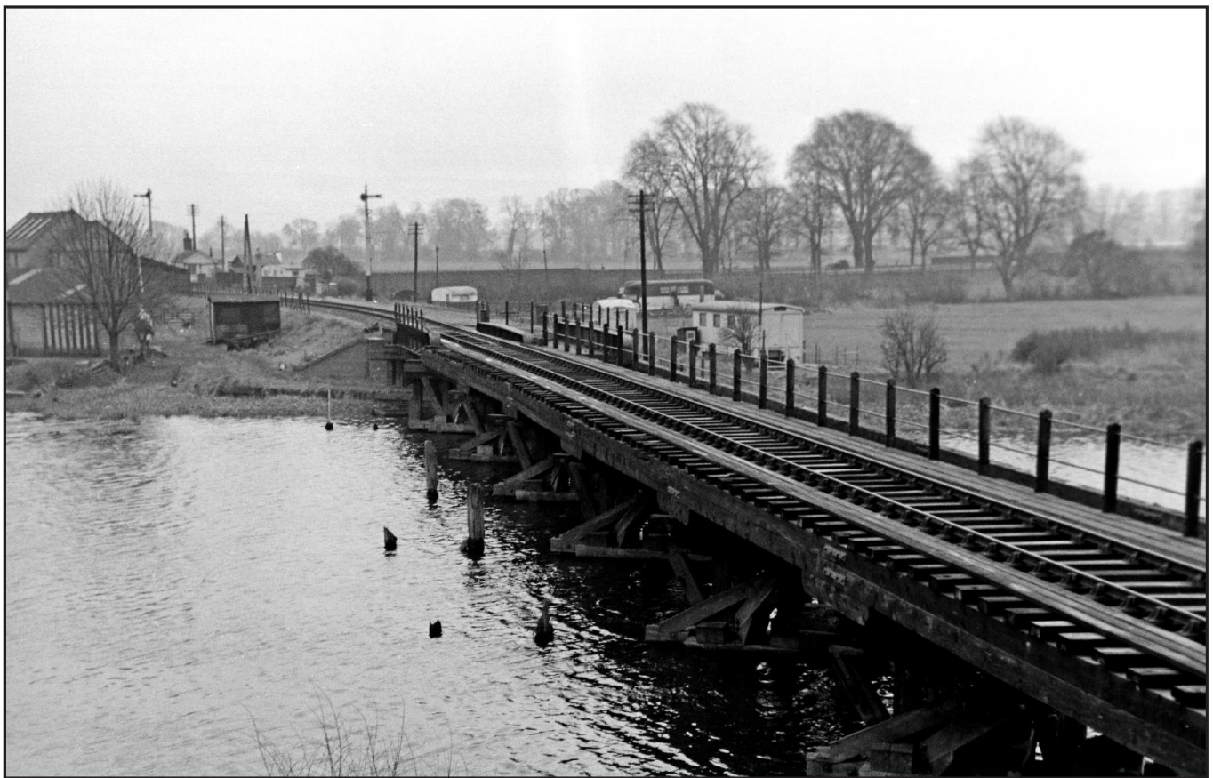
As can be seen from the extract of the Midland Distance Diagrams, the railway between St. Ives and Huntingdon crossed the river Great Ouse no less than six times. Above is the bridge at Godmanchester, taken on 26 th December 1953. The bridge is for single track, but the original was double track, shown by the second iron bridge on the further bank. [Transport Treasury]
