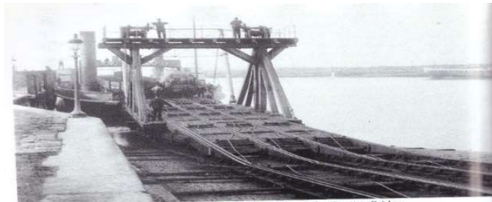
Goods boat PS Ballermic at Granton showing the rails over the Floating Bridge. Kirkcaldy Museum/3324A
