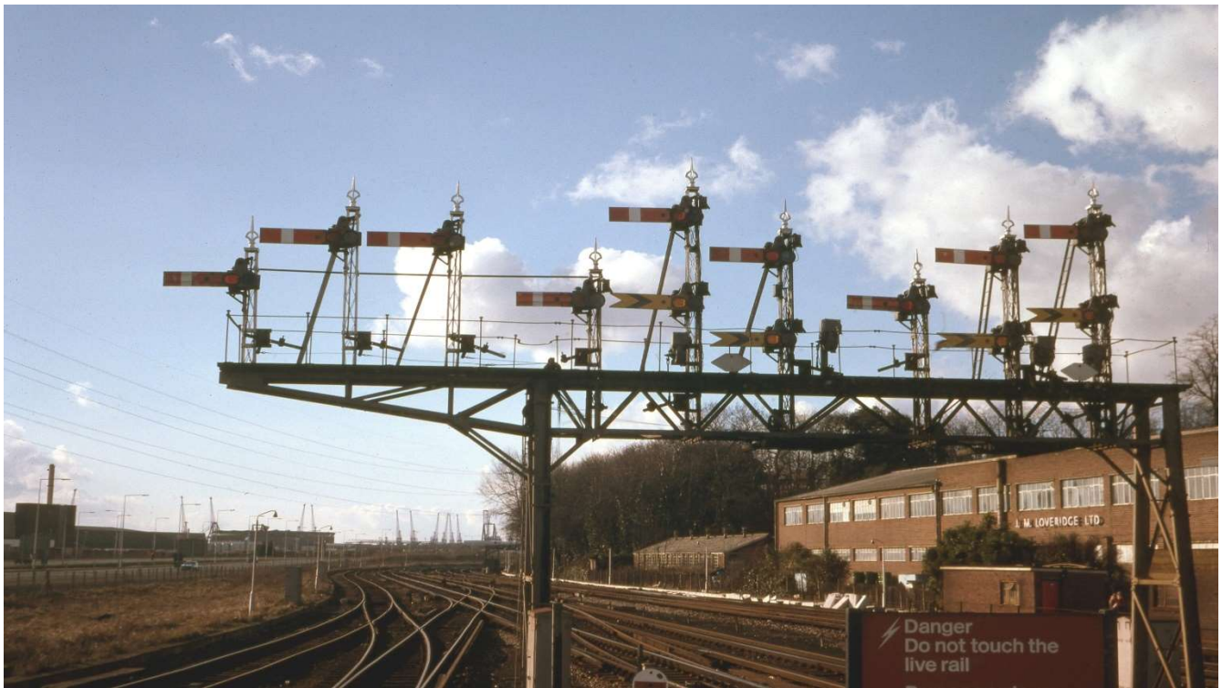
Signalling at the west end of Southampton Central
