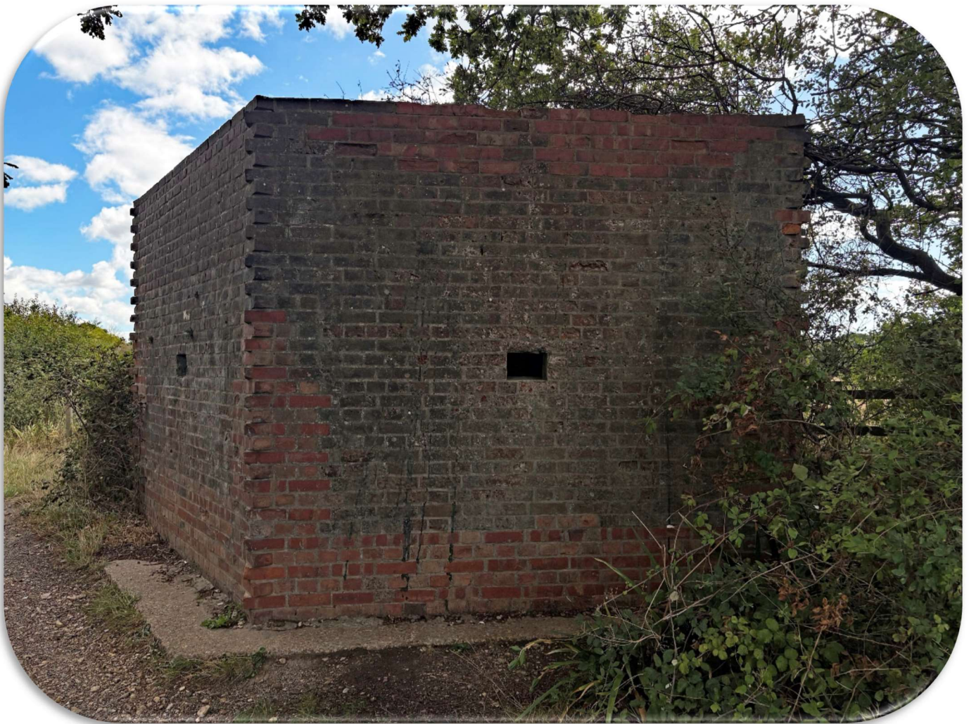
The Pillbox located on the East side of the former line to the South of Hayling North station.
