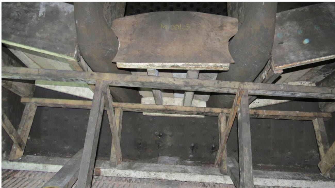
Shuttering in place in firebox, before cement pouring.
