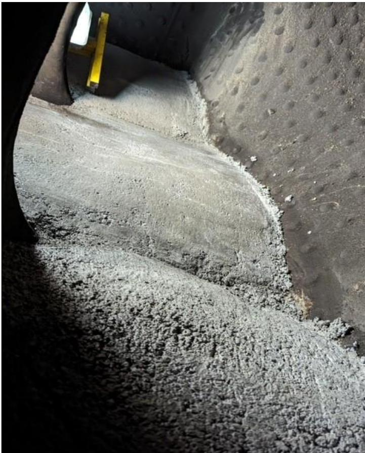
After pouring the upper surface of the arch (in reality there are three arches) it was smoothed to make cleaning easier.
