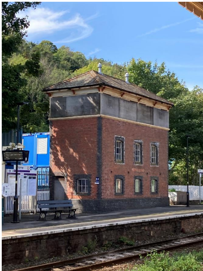
Torre signal box. As with many ex-GWR lines, the wider than usual "6 foot" between the running lines is a legacy of broad gauge days.
