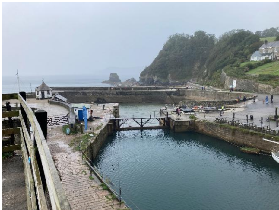
A very wet Charlestown Harbour, near St Austell.
