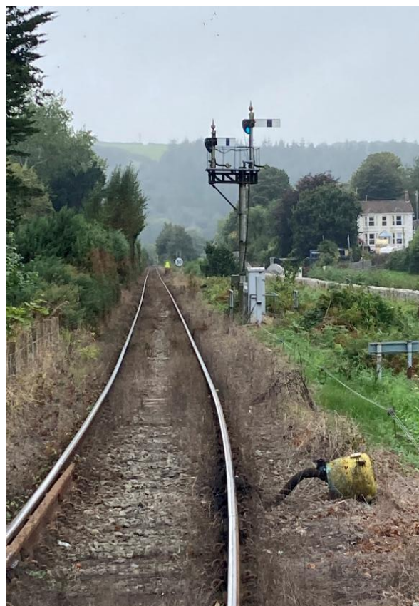
Towards Newquay from Middleway LC, showing the GWR pattern lower quadrant bracket signal. The main signal is for the line to Par station, the junction signal is for the goods line to St Blazey yard, depot and Par Docks. Note the check rail on the curve and the rail lubricator.
