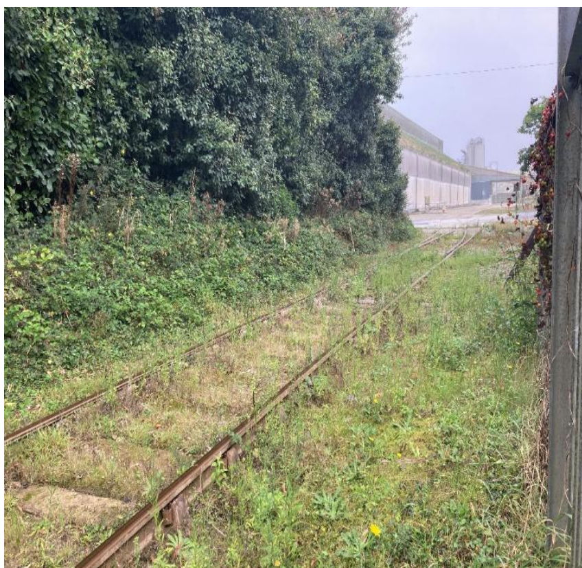
Looking through the fence towards the remaining dockside tracks and facilities inside Par Docks.
