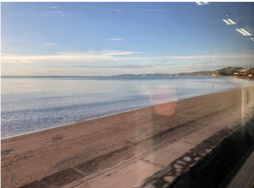
Wednesday morning's view from a Class 165 unit over the recently rebuilt sea wall, heading to Newton Abbot, then Totnes.
